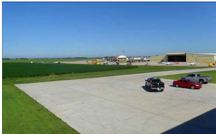
A shot taken from the second floor deck at Spencer Avionics. The spacious concrete ramps at the Spencer airport can be seen in this photo.
